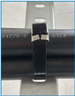
Example of Direct-to-Rung installation.
