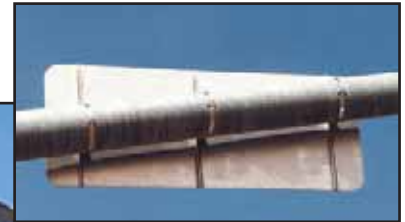
Mast Arm Sign Installation
