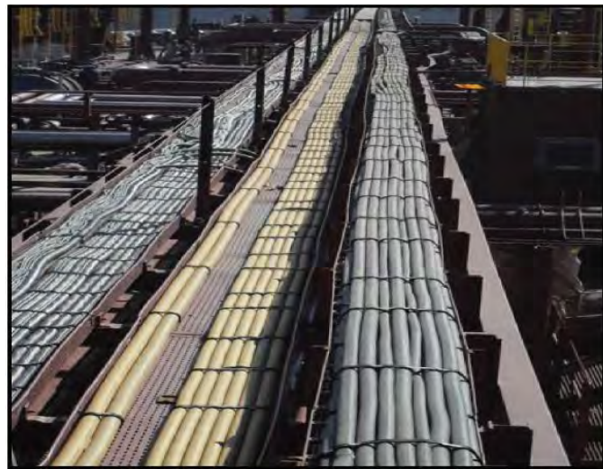
Used in cable management applications to reduce the risk of cutting or abrading cable
